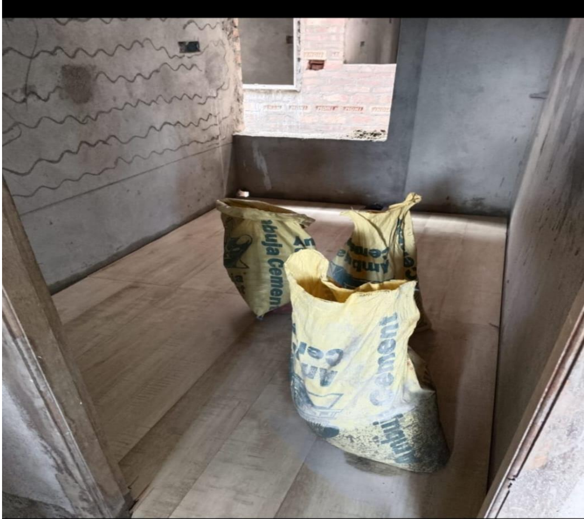
Kitchen floor tiles fitting started.
